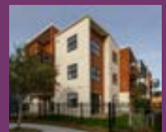
Apartments in the Oranga Development.
