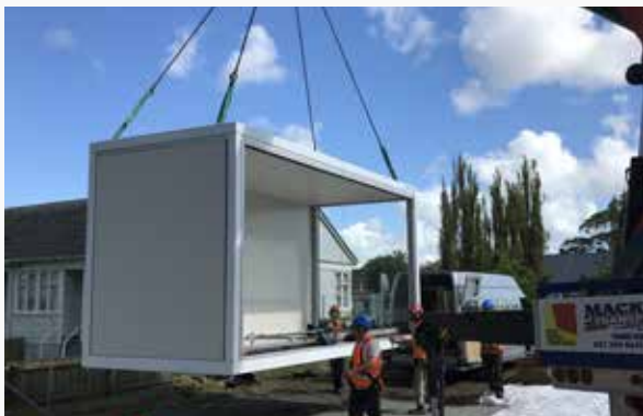
Above: HLC's construction team installing the Information Cube on Hendon Avenue
